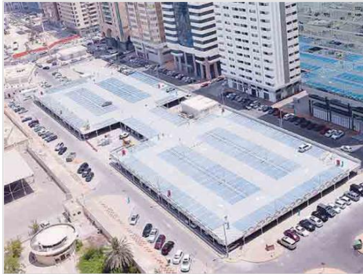
The parking facility, which was completed within a three-month record time, spans over 8,252 square meters and can accommodate 562 vehicles.— Courtesy photo
